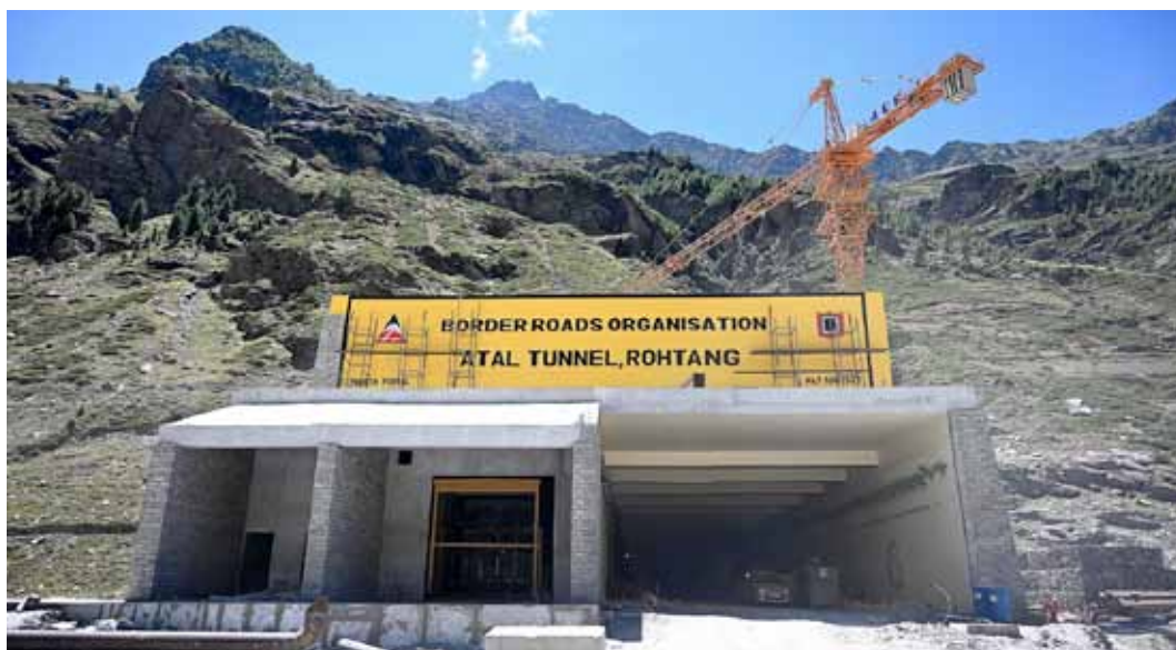
Top: Construction team members work inside the Atal Tunnel near Solang in Himachal Pradesh. This photograph was taken on September 1, 2020; Left: The north portal of the Atal Tunnel, captured on September 1, 2020
